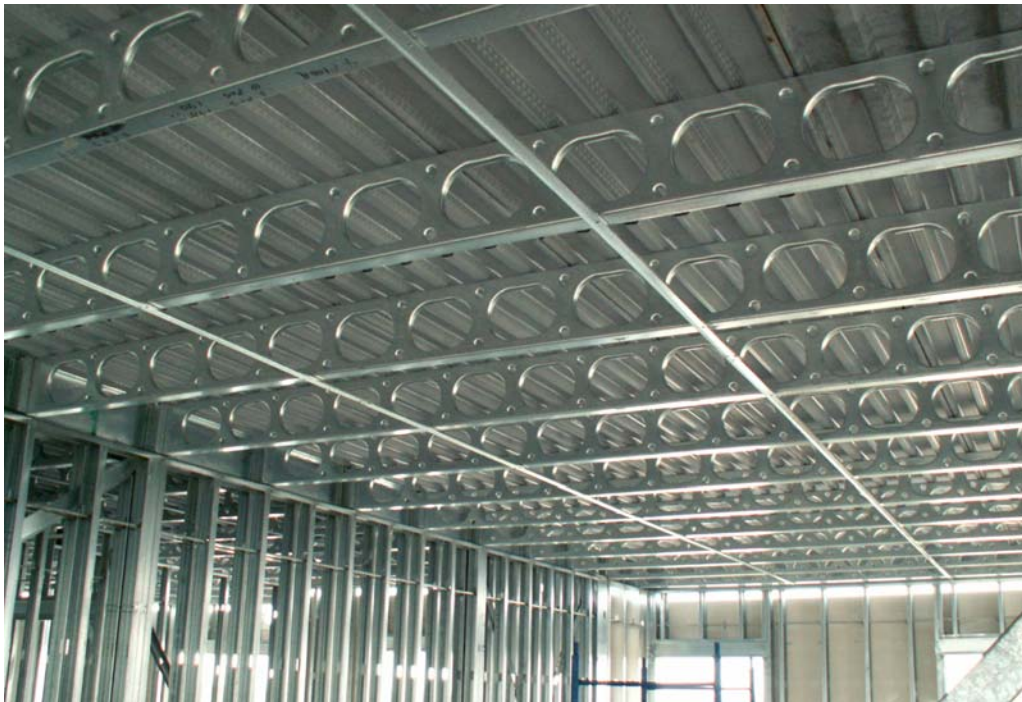
Lightweight MegaJoist provides the strength needed for this concrete-on-steel decking floor system.
