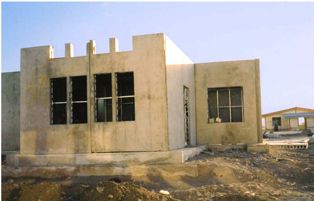
This single-story residence is quickly erected using ThermAlloy Precast Panels.
